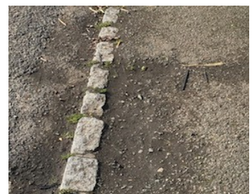
Kerb to footway of granite setts
